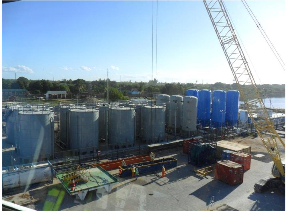
*Figure 3-10 Mtwara Port. Container being loaded onto supply vessel in the foreground. Mud plant and storage in the background. (Source: COWI).*
