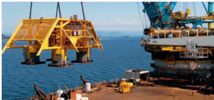
The subsea installation on Tordis will extend the field's producing life and improve recovery.
